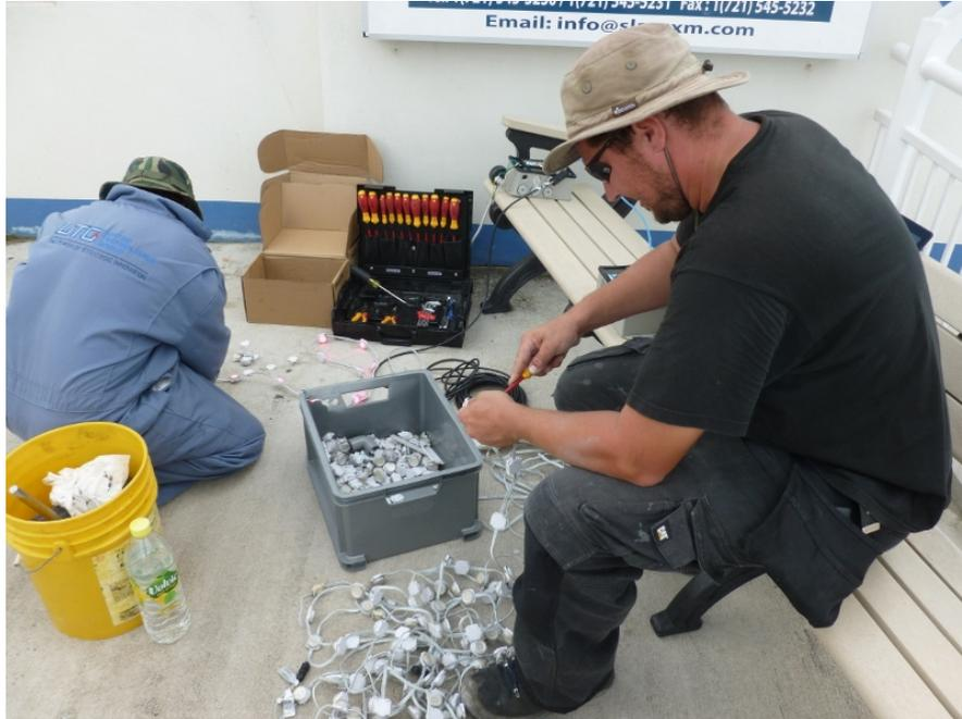
**PHOTO OUTLINE:** Two technicians at work on the Causeway LED lighting system.
